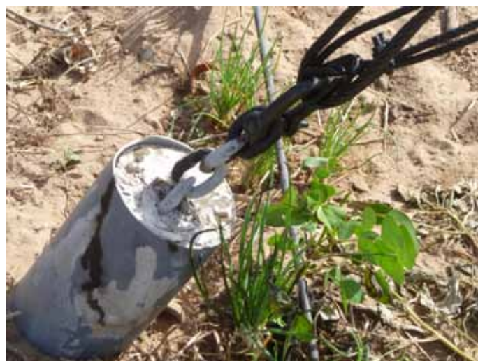
Fig. 5: Chain poured into concrete
