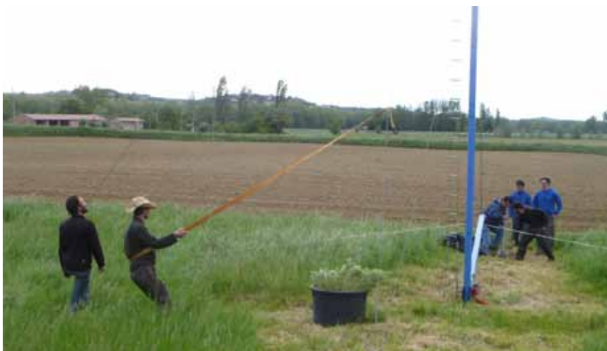
Fig. 14: Pulling top guy wire strap
