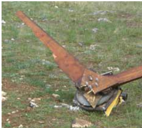
Fig. 64: Loss of balancing weight
