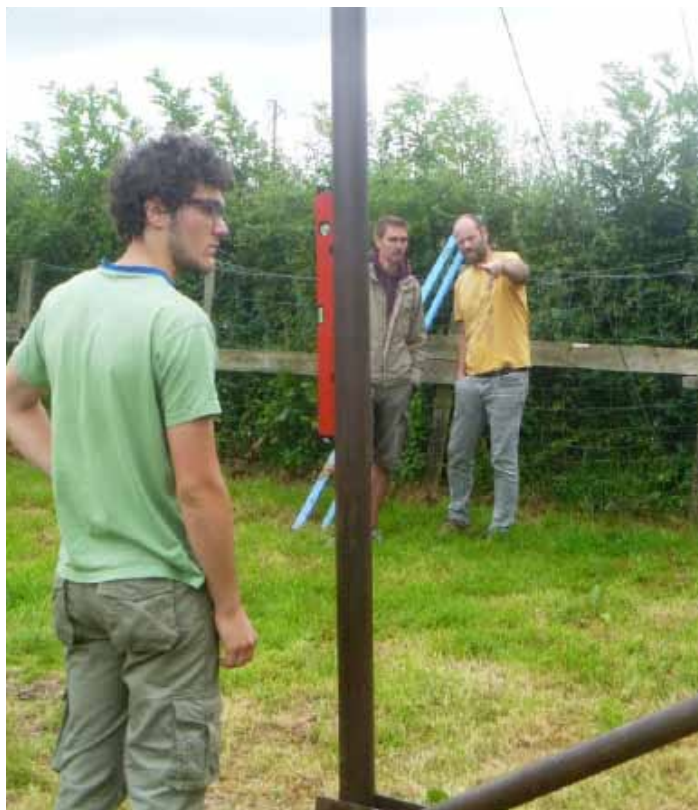
Fig. 24 : Verticality check at the bottom of the tower
