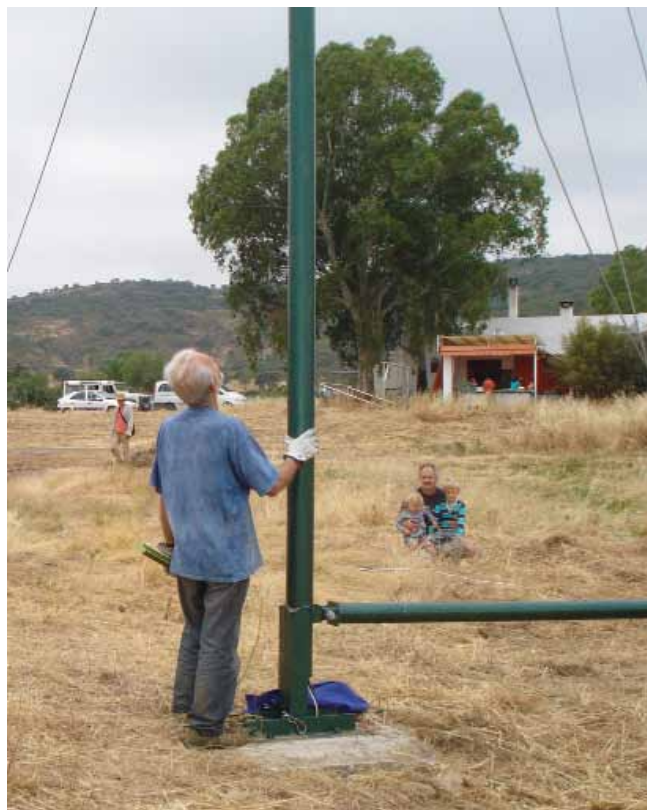
Fig. 25 : Verticality check of the upper parts of the tower
