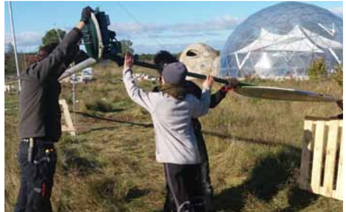
Fig. 20: Installing the tail
