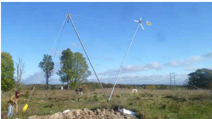
Fig. 15: Lowering the tower
