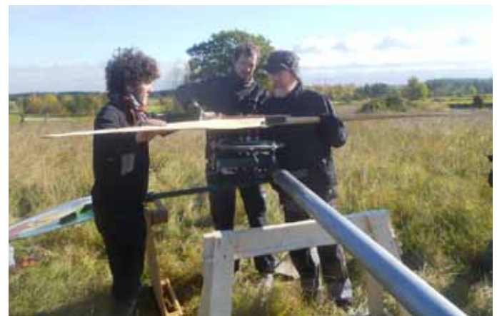
Fig. 21: Installing the blades
